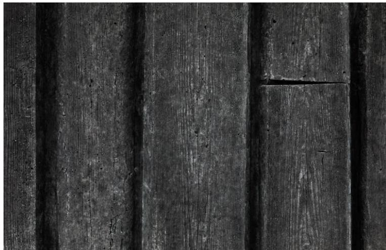
The concrete, which is colored with black iron oxide pigments of LANXESS' proven Bayferrox brand, reproduces the weathered material wood.
