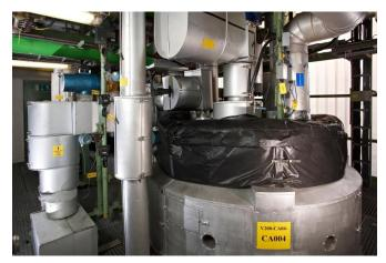
A high-pressure Hastelloy C4 autoclave with a capacity of five cubic meters designed for reaction pressures up to 250 bar and reaction temperatures up to 230 °C at Saltigo's designated hydrogenation plant at its Leverkusen site. Photo: Saltigo GmbH
